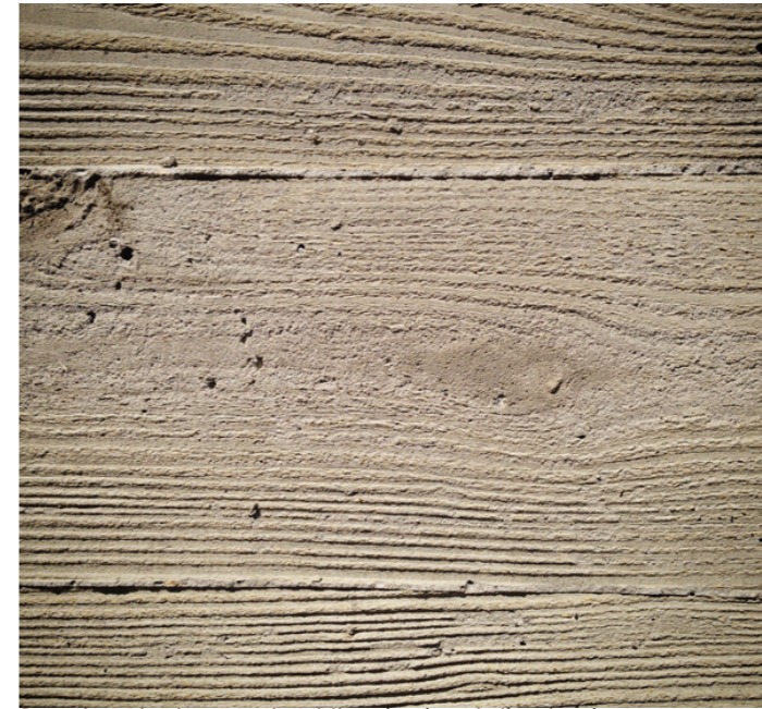
Board marked concrete at the viewing station to give a natural effect
