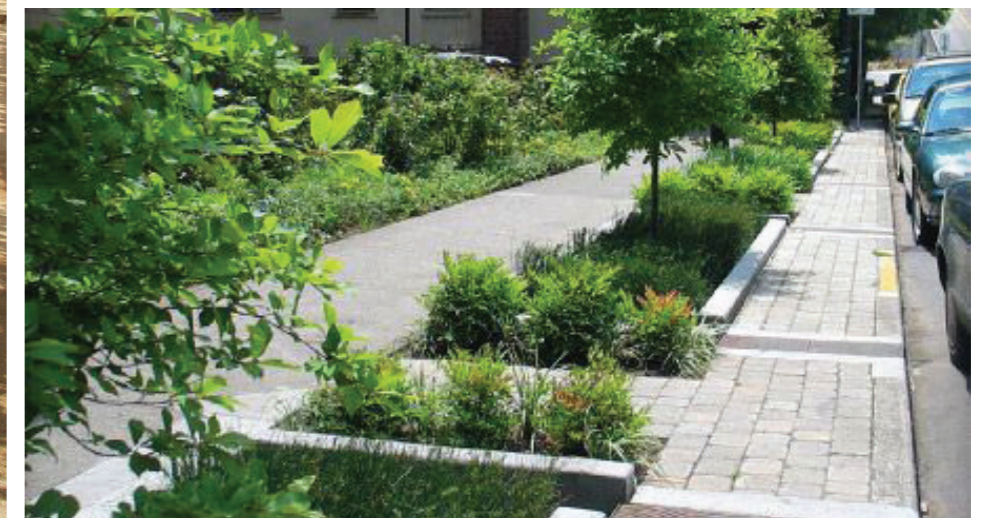
Green streets with water attenuation opportunities offer a smart solution for water drainage while creating green corridors for wildlife
