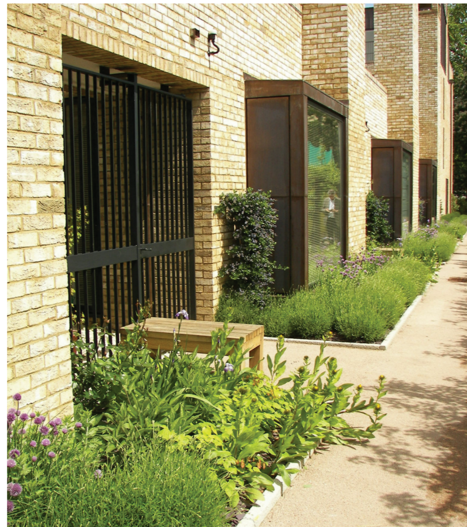
Soft treatment of the facades provides privacy screening and clear separation between public and private
